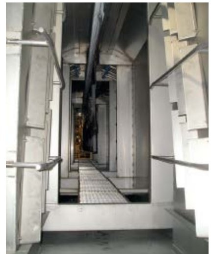
Washing, degreasing, drying and blasting of parts
